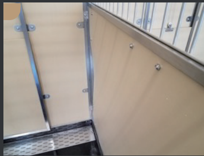
Side wall: stainless steel frame and HDPE panel
