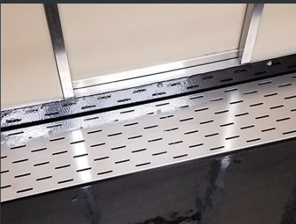
Filter cover for protecting the drainage trough
